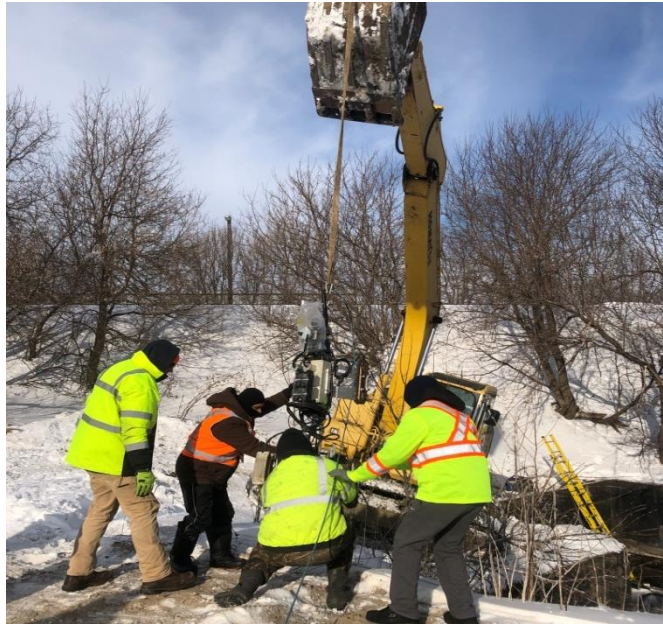
Figure 4. Surveyor deployment in the RC pipe
